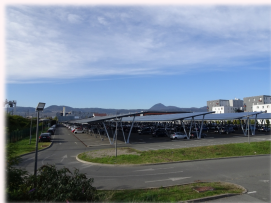
Ombrières CHU Estaing – Clermont-Ferrand
